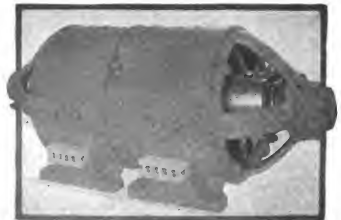
Fig. 8—Motor-generator set by General Electric Company
